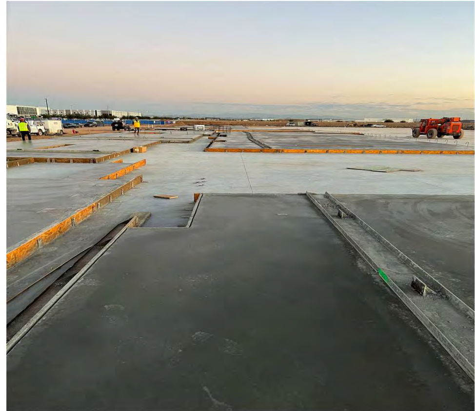
_Tilt-Up Panels_ 4000 psi and 5000 psi with Natural Pozzolan.
