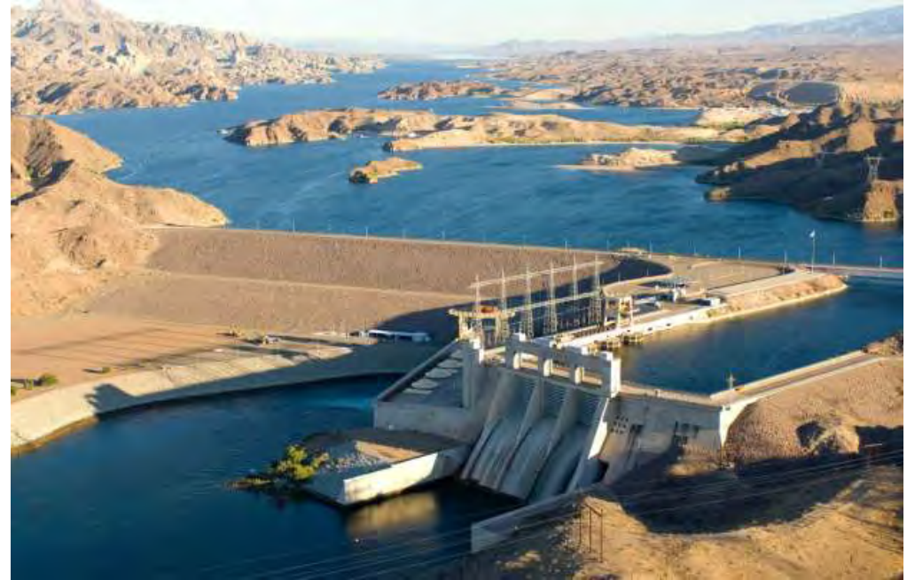
Davis Dam (AZ/NV)- Utilization of Natural Pozzolan as SCM in Mass Concrete.
